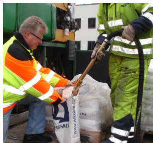
Ejector filling of bead tank
