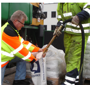
Ejector filling of bead tank
