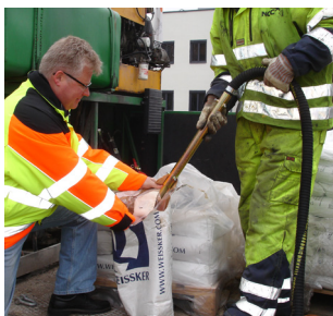
Ejector filling of bead tank
