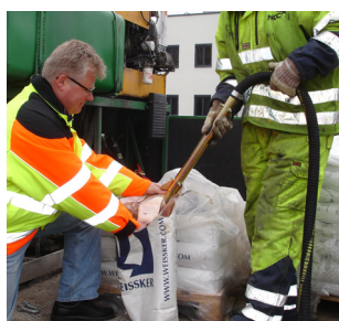
Ejector filling of bead tank
