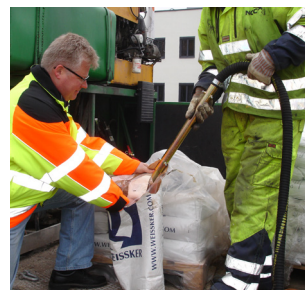
Ejector filling of bead tank
