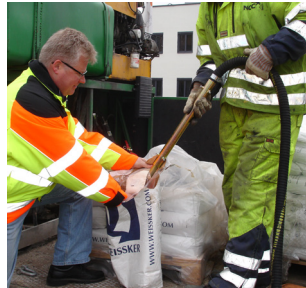
Ejector filling of bead tank
