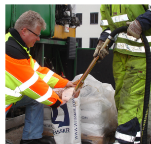
Ejector filling of bead tank
