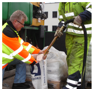
Ejector filling of bead tank
