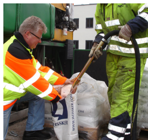
Ejector filling of bead tank
