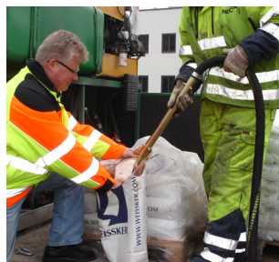
Ejector filling of bead tank
