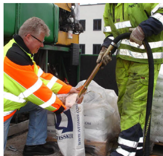
Ejector filling of bead tank
