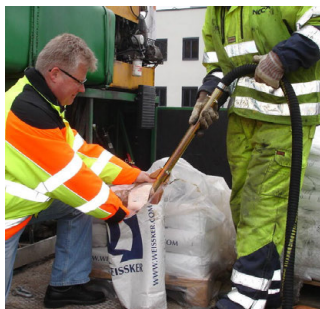
Ejector filling of bead tank
