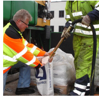
Ejector filling of bead tank
