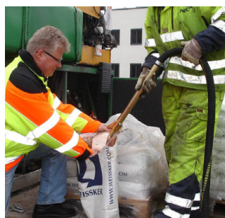
Ejector filling of bead tank
