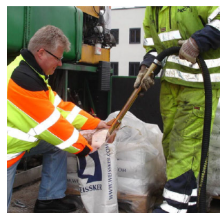
Ejector filling of bead tank
