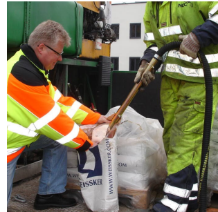
Ejector filling of bead tank
