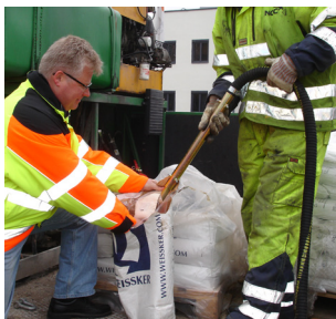
Ejector filling of bead tank
