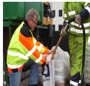
Ejector filling of bead tank
