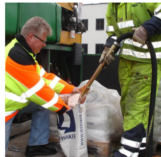
Ejector filling of bead tank
