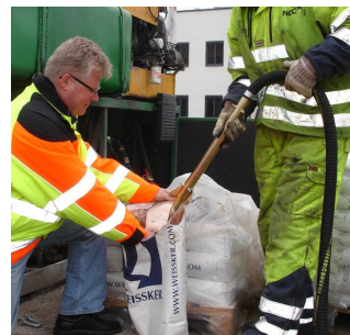
Ejector filling of bead tank
